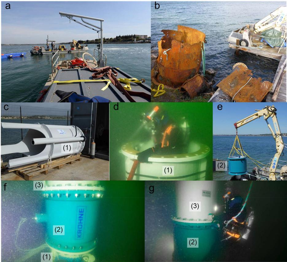
**Fig. 5.** Collection of the different views taken during the stages of the installation site. (a) placement of the barges directly above the spring. (b) view of the old metal nozzle that was present on the submarine spring. (c) view of the lower part (flow collector, 1) of the new device. (d) view of a diver installing the water collector on the underwater spring. (e, f) view of the electromagnetic flowmeter(2). (g) view of the stilling tube (3) installed above the flowmeter (2).
