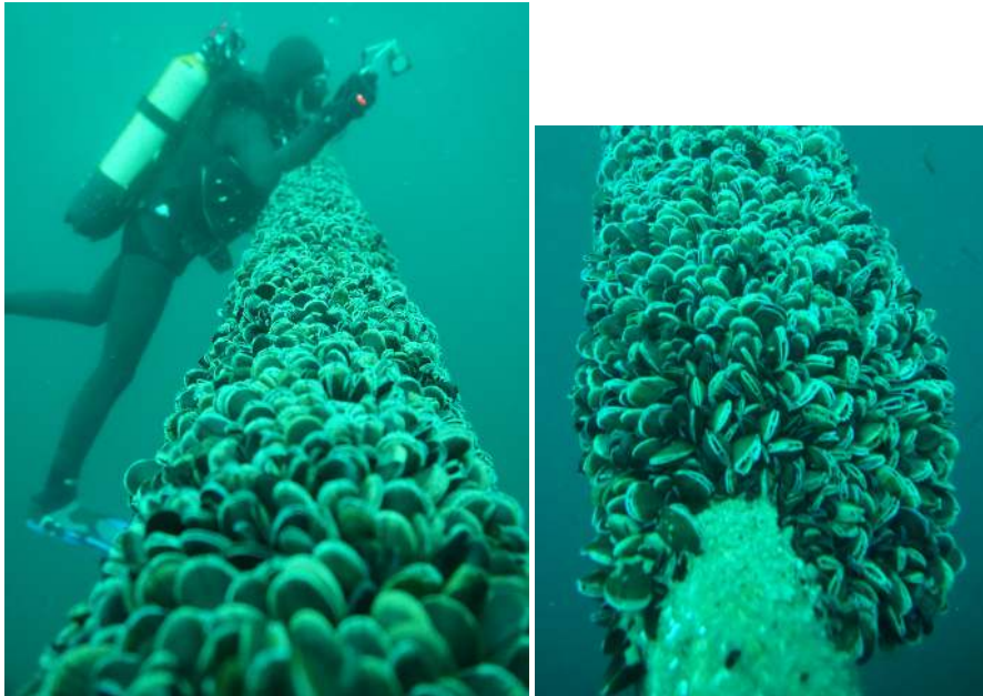
Figure 1: Illustration of mussel colonisation on a mooring line (West coast of France on a 0.1m diameter mooring line at 10m depth) [15].
