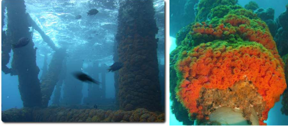
Figure 2: Illustration of corals colonisation on a jacket of marine platform in West Africa, with a tubular bracing structure of 0.2 to 2m diameter.
