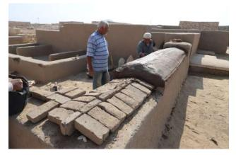
Figure 9: Rounded shape forming the protective capping prepared with bricks and two coats of plaster finish.
