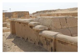
Figure 6: The conservation works (method C) did not prove efficient during the 2020 rains.  ${}^{\circ}$  T. Joffroy
