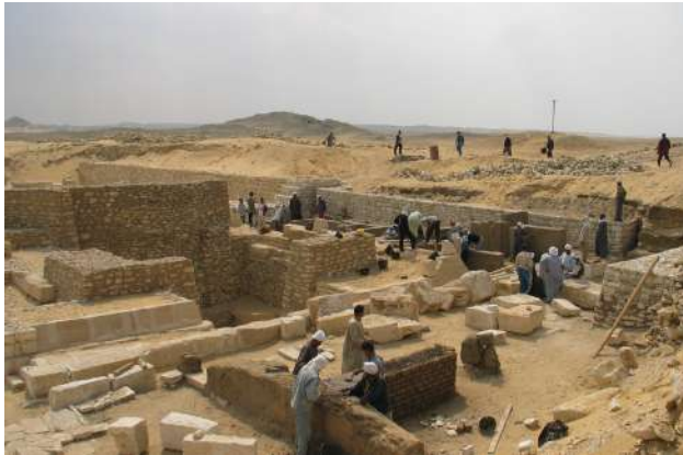
Figure 5: Conservation works on the mudbrick structures (methods A and B).
