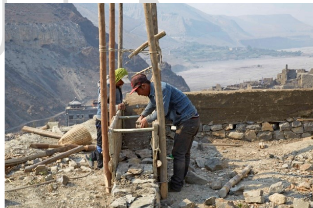
Rammed earth masonry walls under construction, Kagbeni, Lower Mustang, 2016— ©Marie Schuiten
