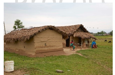
Clearly separated roofs, the use of "open" materials (thatch or tiles) reduce wind forces, and thus the risk of roof blow-off, Tharu village, Terai, 2016. –©Marie Schuiten
