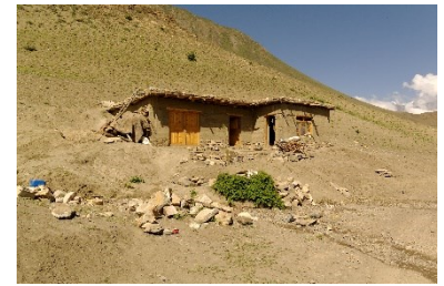
House between Muktinath and Kagbeni. The shape of the house, embedded in the slope, limits the risks of landslides and avalanches, thus offering an optimal facade facing the sun and a minimum of other openings. 2013– ©Mathilde Chamodot
