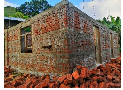
Brick in cement mortar masonry, Halesi Tuwachung, Khotang, 2018 – ©HRRP
