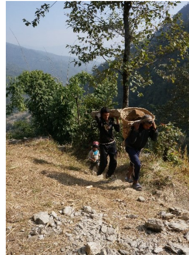
The extraction and transport of local stone, sand and soil for the construction of stone walls has a very low energy demand, although it is labour intensive, Magapauwa, 2016 –©CRAterre
