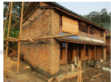
Retrofit demo house, Annapurna rural municipality, 2019 – HRRP©
