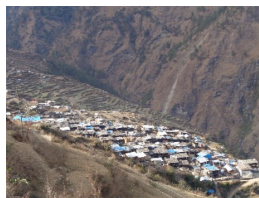
Compact row-housing, Gatlang, Rasuwa, 2016 – ©CRATerre
