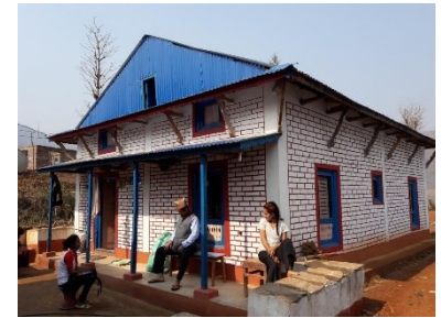
Load Bearing stone masonry in mud mortar; Location Sunkoshi Rural Municipality-06, Sindhuli, 2018 – ©HRRP
