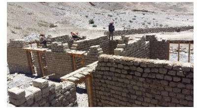
Demo house construction in Dhye, Mustang, 2016 – ©FAP
