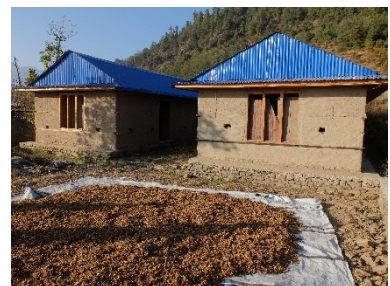
Heavy rains protection. Raised ground floor on a large platform, Sindhupalchok 2018 – ©CRAterre
