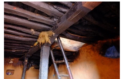
Burnt wood structure: this process protects the surface of the wood and slows the spread of fire, Dolakha, 2015 – ©CRAterre
