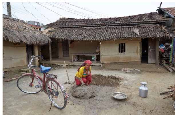
Mud plaster preparation, for wattle & daub house maintenance, Tharu village, Terai, 2016— ©Marie Schuiten
