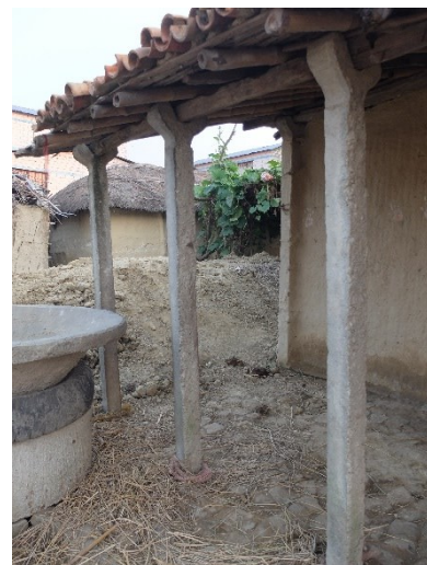
Floods protection. RCC post, Terai 2022 – ©CRAterre
