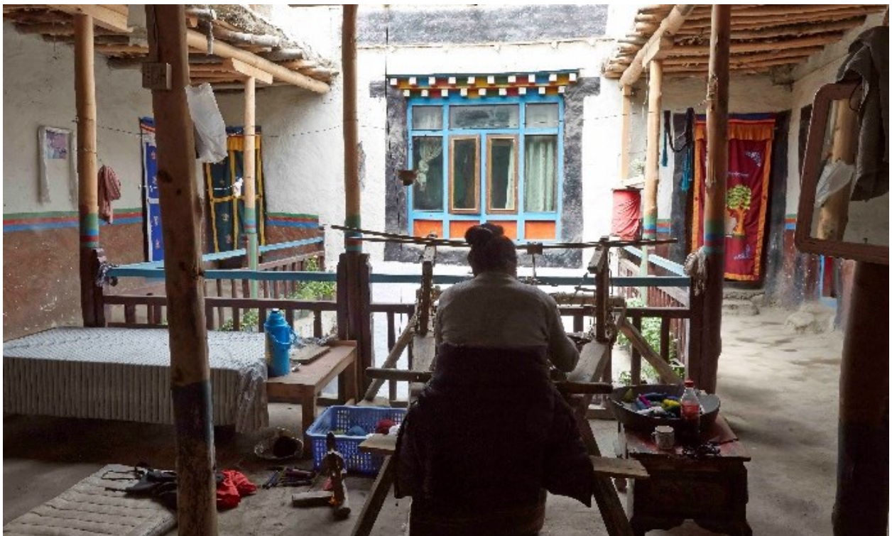
Courtyard house, used as a workshop, and other domestic uses, Tsarang Village, Upper Mustang, 2016 – © Marie Schuiten
