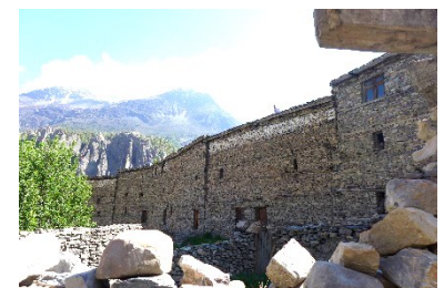
Settlement in the village of Manang. Minimum openings in massive stone walls, 2013– ©Mathilde Chamodot
