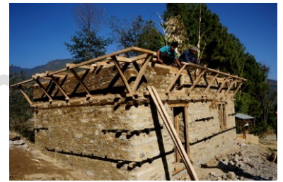
Demo house construction in Magapauwa, Dolhaka, 2016 – ©CRAterre
