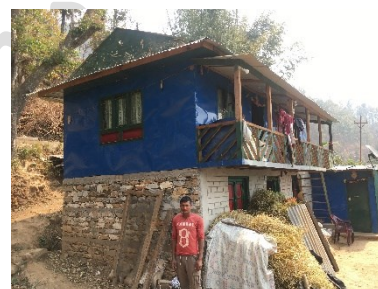
Hybrid structure, Timber and CGI fencing on masonry ground floor, Molung, Okhldunga. ©HRRP
