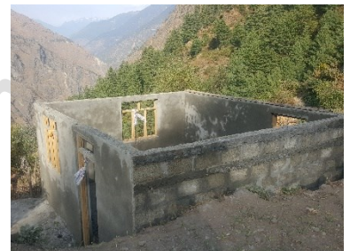
Hollow concrete blocks in cement mortar masonry, Naukunda-rural-municipality, Rasuwa-, 2018 – ©HRRP
