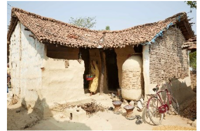
Ventilation, humidity and temperature are regulated through the use of heavy, breathable materials (earth) and light woven materials (bamboo), Mithali village, Terai, 2016 –©Marie Schuiten
