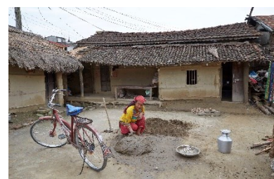
Artisan preparing mud mortar for regular maintenance of the plasters, Mithali village near Janakpur, 2016– ©Marie Schuiten
