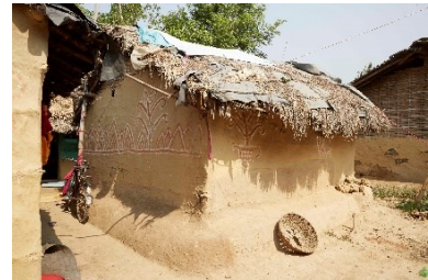
Flood protection. The basis of the walls is surrounded by a mud layer, which is cyclically eroded and repaired. Terai, 2016 – ©Marie Schuiten
