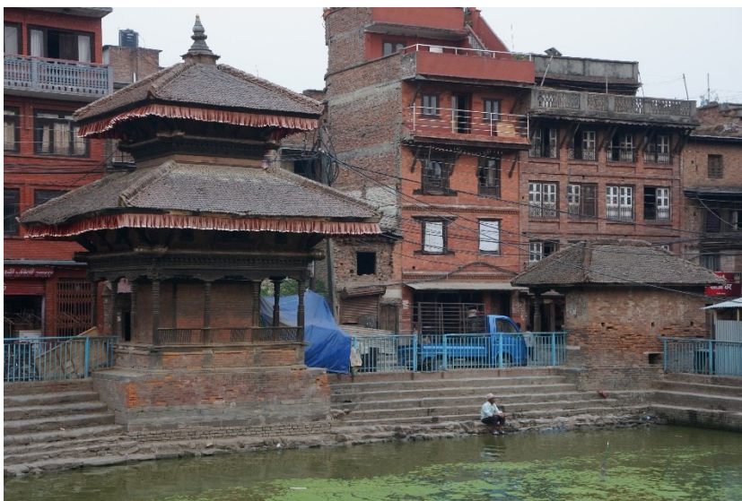
Vertical extensions and hybridation of the building typologies, Patan 2016 – © CRAterre
