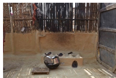
Timber and bamboo protected from fire with mud plasters, Mithali village, Terai, 2016– ©Marie Schuiten
