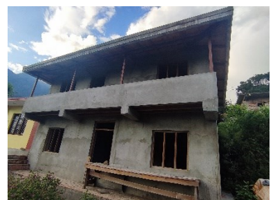
Hollow concrete blocks in cement mortar masonry, Sindupalchowk, 2017 – ©CRAterre
