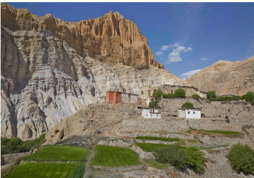
Stone retaining walls consolidating the field and settlement terraces ©Marie Schuiten
