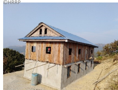
Safe hybrid structure: masonry ground floor & timber storey, Sindhuli. ©HRRP
