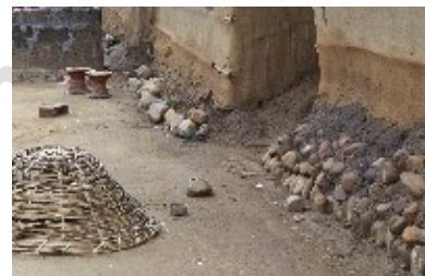
Floods protection. Plinth protected with stones. Tharu village, Terai, 2016 – ©Marie Schuiten
