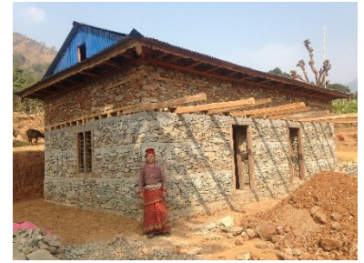
SMM house with light gable wall, 2018– ©HRRP
