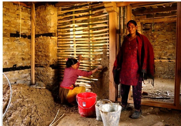
Wattle and daub partition wall, Dolakha, 2016 – ©CRATERre
