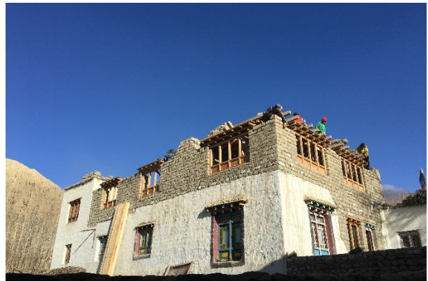
Adobe masonry walls under construction, upper Mustang, 2018 – ©HRRP
