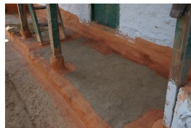
Mud plasters for floor finishing, Dolakha, 2016 – ©CRAterre
