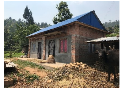
Brick in cement mortar masonry, Lisankhupakhar-rural-municipality, Sindhupalchowk, 2019 – ©HRRP
