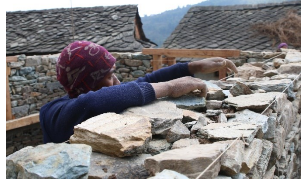
Stone masonry walls, stone slates, Ramechhap, 2017—©HRRP
