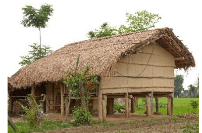
Cross ventilation, bottom ventilation and thick fiber roofing regulate the indoor humidity and temperature , Tharu village, Terai, 2016– ©Marie Schuiten
