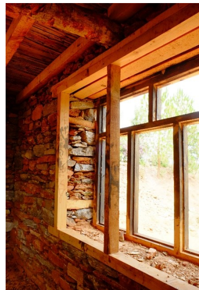
Window frame built as a box, SMM house, Dolakha, 2015 — ©CRAterre
