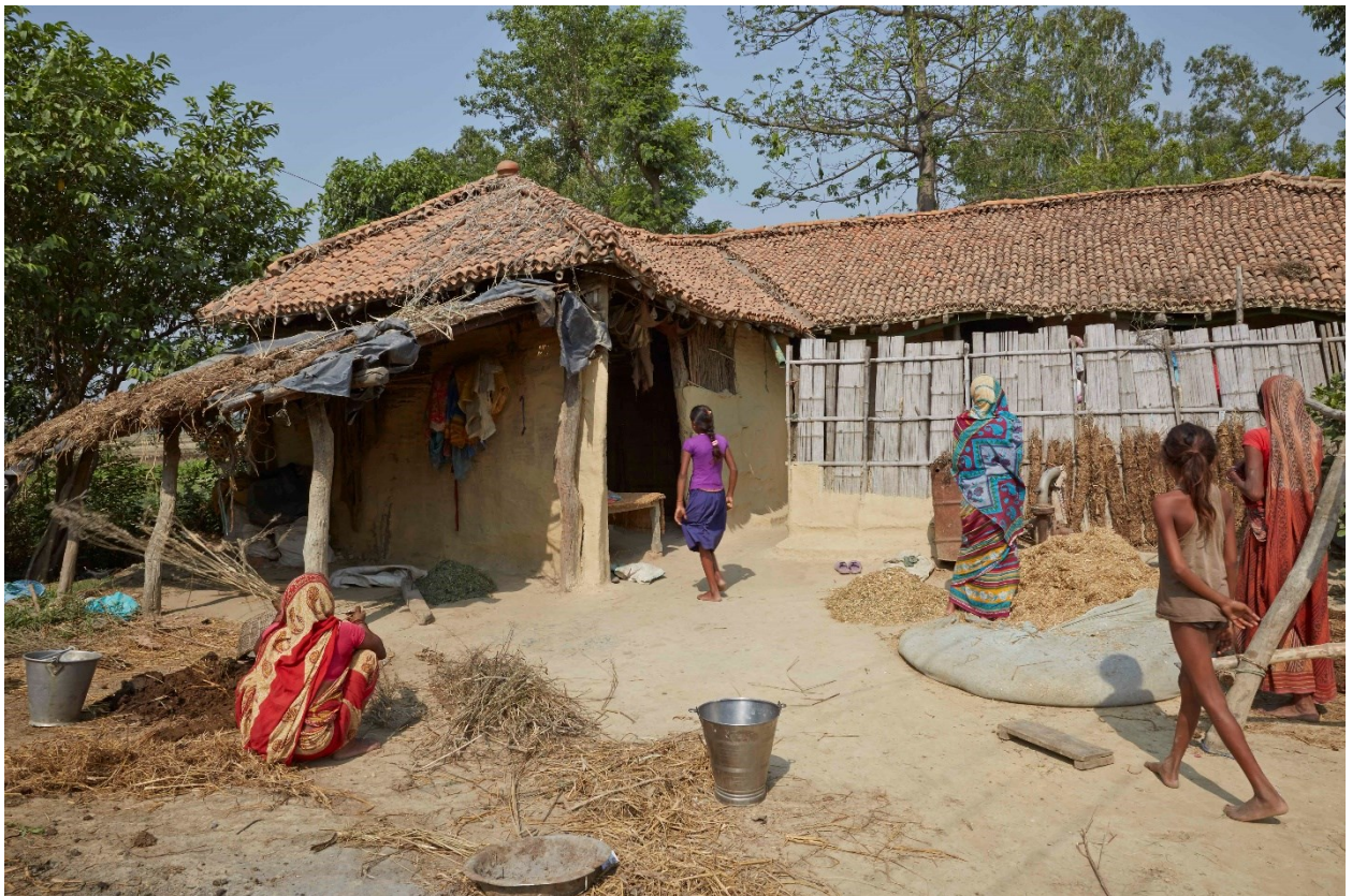
Wattle & daub house, courtyard space, Mithali village, Terai 2016 ©Marie Schuiten
