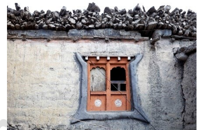
Flat roof used for wood storage, Kagbeni, Lower Mustang, 2016 – © Marie Schuiten
