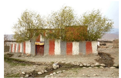
The boundary walls of the plots, made of stones and/or mud bricks, and the maintained vegetation, increase the protection of the buildings. Tsarang village, Upper Mustang, 2016– ©Marie Schuiten
