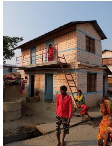
Compressed stabilized earth blocks masonry house, reconstruction program, Lumanti. Simara, Terai, 2022– ©CRAterre
