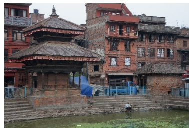
“Fake” traditional “Newari façade- the façade is “plugged on a Brick masonry and RCC frame building, Bhaktapur, 2016 ©CRAterre
