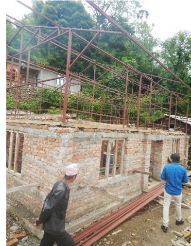
Light steel frame structure for upper storey on BMC ground floor, Jiri, Dolakha, 2017 – ©HRRP
