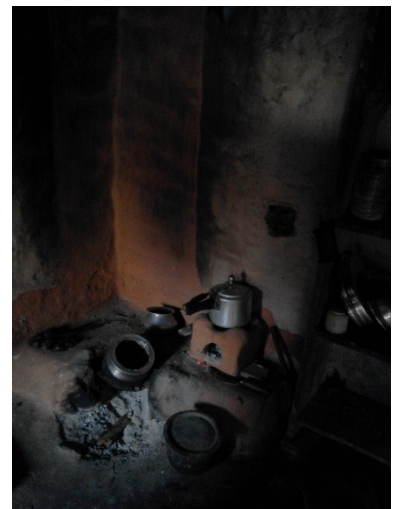
Effects of smoke on the interior walls of a kitchen, where firewood is used on an open fire, with no chimney to vent the smoke– ©CRATERRE
