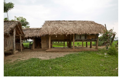
Timber house on stilts, Tharu village near Sauraha, Terai 2016 ©Marie Schuiten
