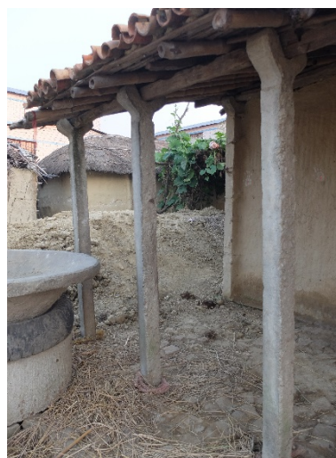
Floods protection. RCC post, Terai 2022 – ©CRATERRE
