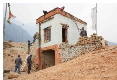
Roof maintenance, adobe house with clay plasters /paints. Drakmar, Upper Mustang 2016 – ©Marie Schuiten
