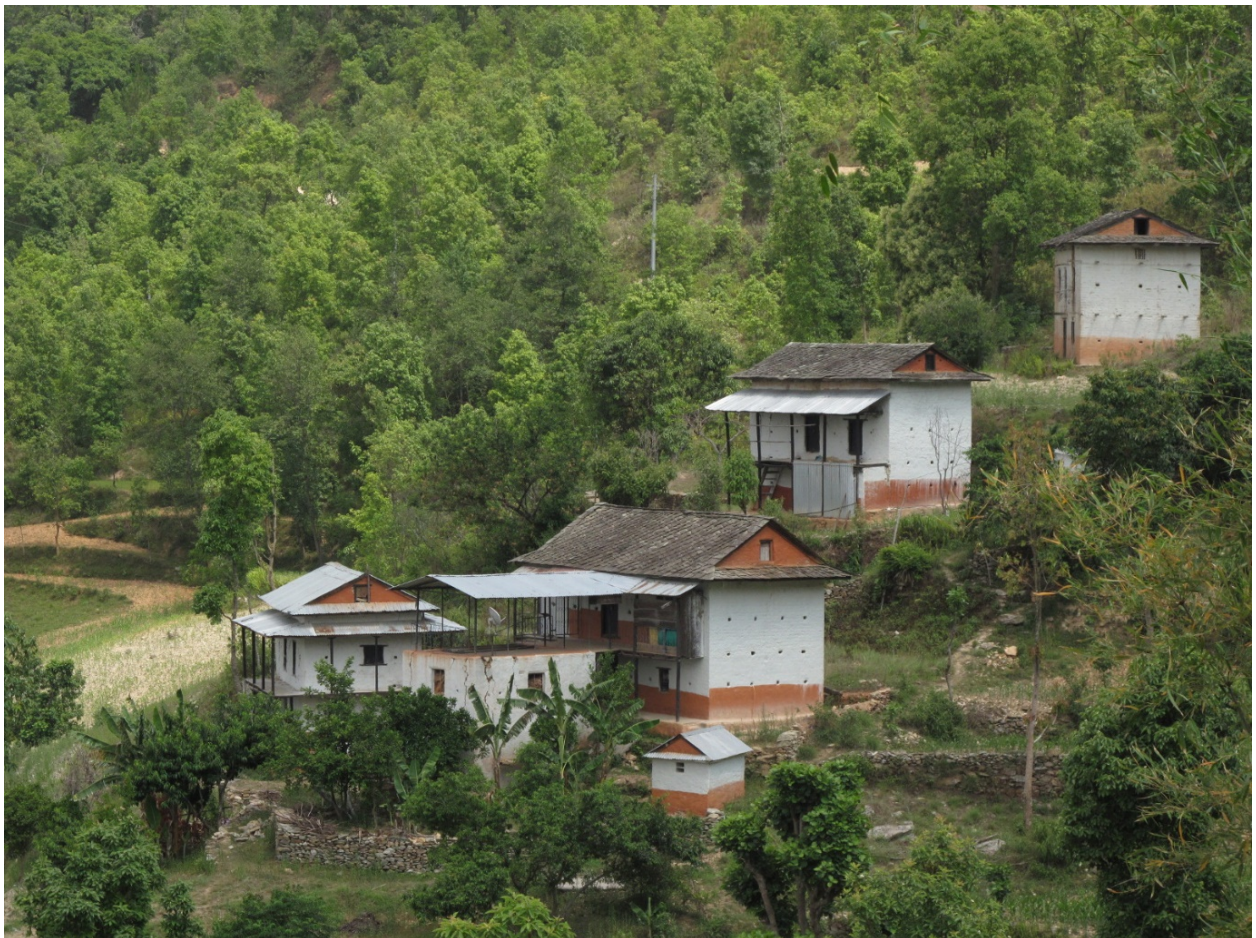
Cluster of houses, Dolakha, after 2015 Gorkha’s earthquake –©CRAterre
