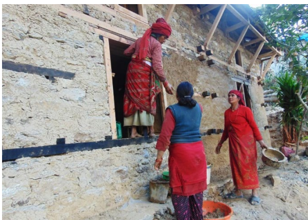
Mud plasters application on SMM house, Dolakha, 2016 – ©CRAterre
