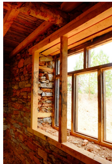
Window frame built as a box, SMM house, Dolakha, 2015 – ©CRAterre
