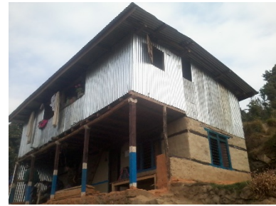
Sound hybrid structure: masonry ground floor & timber+ CGI sheets storey, Bhojpur. ©HRRP
