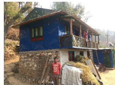
Hybrid structure, Timber and CGI fencing on masonry ground floor, Molung, Okhldunga. ©HRRP
