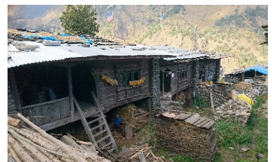
CGI sheets roofing in place of wooden tiles, in cold areas reduces indoor temperatures, Gatlang, Rasuwa –©HRRP
