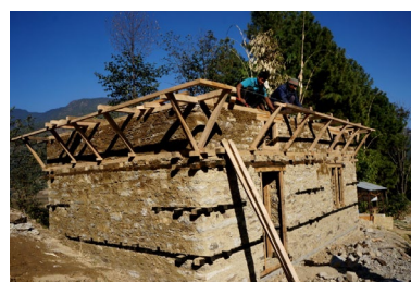
Demo house construction in Magapauwa, Dolhaka, 2016 – ©CRAterre
