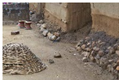
Floods protection. Plinth protected with stones. Tharu village, Terai, 2016 – ©Marie Schuiten
