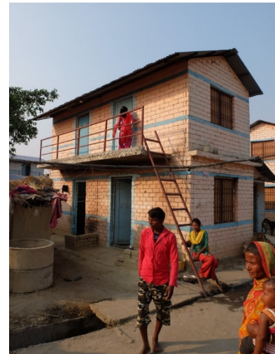
Compressed stabilized earth blocks masonry house, reconstruction program, Lumanti. Simara, Terai, 2022– ©CRAterre
