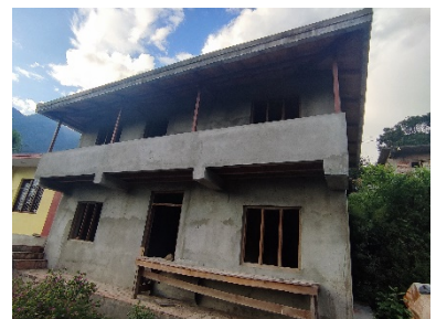
Hollow concrete blocks in cement mortar masonry, Sindupalchowk, 2017 – ©CRAtterre
