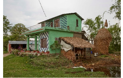
Brick masonry house, Tharu village near Sauraha, Terai 2016 ©Marie Schuiten
