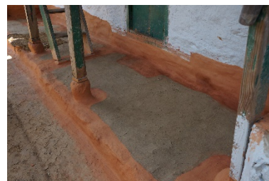
Mud plasters for floor finishing, Dolakha, 2016 – ©CRAterre
