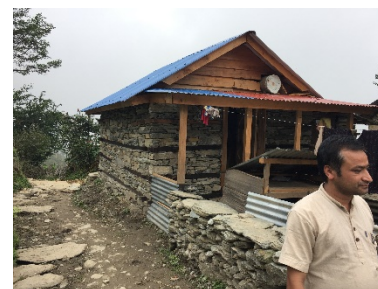
Clear dissociation of roof and veranda for better roof behaviour in case of strong winds, Dadhing 2018 –©HRRP
