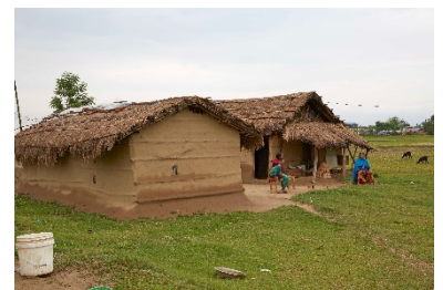
Clearly separated roofs, the use of "open" materials (thatch or tiles) reduce wind forces, and thus the risk of roof blow-off, Tharu village, Terai, 2016. –©Marie Schuiten
