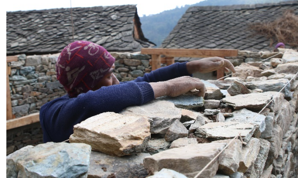
Stone masonry walls, stone slates, Ramechhap, 2017—©HRRP
