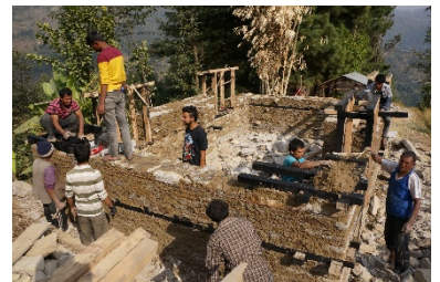
Training for masons, under engineers supervision: in a large proportion, men benefit from these opportunities, 2017, Dolakha– ©CRATERRE
