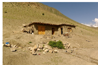
House between Muktinath and Kagbeni. The shape of the house, embedded in the slope, limits the risks of landslides and avalanches, thus offering an optimal facade facing the sun and a minimum of other openings. 2013– ©Mathilde Chamodot
