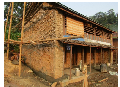
Retrofit demo house, Annapurna rural municipality, 2019 – HRRP©
