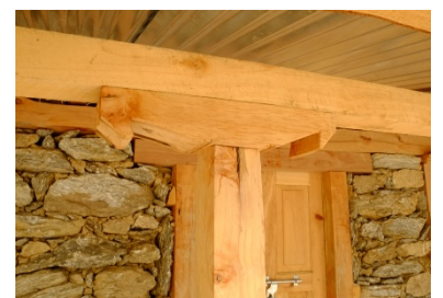
Capital for the support of timber beams, allows lateral displacements without structural disorder, Dolakha, 2105– CRAterre©
