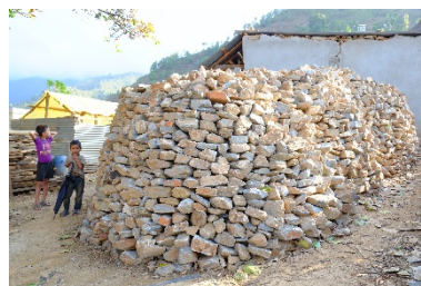
Salvage of stones from damaged constructions, Dolakha, 2015– ©CRAterre
