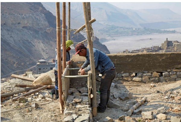
Rammed earth masonry walls, Upper Mustang, 2016 – ©Marie Schuiten
