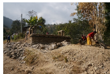
The extraction and transport of local stone, sand and soil for the construction of stone walls has a very low energy demand, although it is labour intensive, Magapauwa, 2016 –©CRAterre
