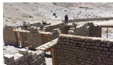
Demo house construction in Dhye, Mustang, 2016 – ©FAP
