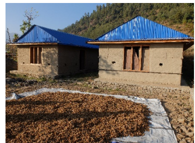
Heavy rains protection. Raised ground floor on a large platform, Sindhupalchwok 2018 — ©CRAterre
