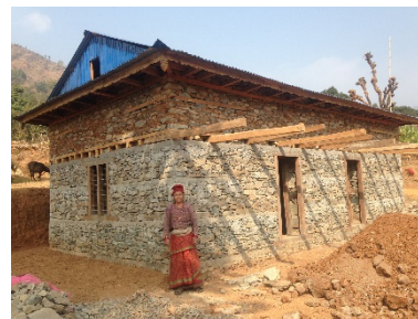
SMM house with light gable wall, 2018– ©HRRP
