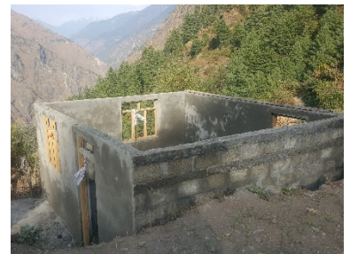
Hollow concrete blocks in cement mortar masonry, Naukunda-rural-municipality, Rasuwa-, 2018 – ©HRRP
