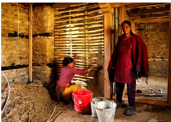
Wattle and daub partition wall, Dolakha, 2016 – ©CRAterre
