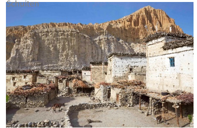
Access to the courtyard houses, Tetang, Upper Mustang, 2016 – © Marie Schuiten
