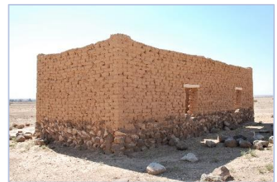
Simple house – adobe walls with stone plinth – © CRAterre
