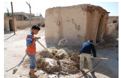
Preparing mud plaster – © CRAterre
