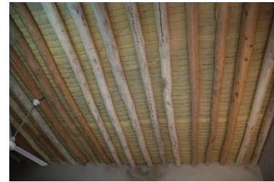
Ceiling sealing course made with woven polypropylene – © CRAterre
