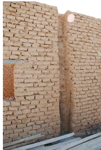
Vertical recesses in adobe wall for pouring reinforced concrete pillar – © CRAterre
