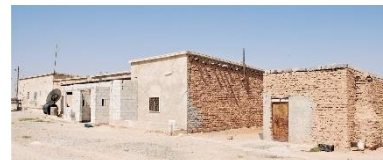
Concrete slabs and cement plasters over adobe load-bearing walls – © CRAterre
