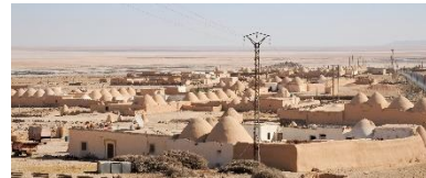
Courtyard earthen dome houses, Aleppo gov. – © CRAterre
