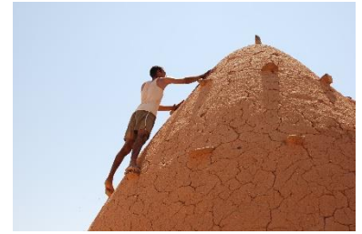
Maintenance: replastering – © CRAterre
