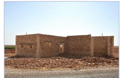
Simple house – stone walls – © CRAterre
