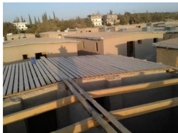
Al-Faroukia - construction site: adobe masonry (left); roofing (middle); plastering (right) – © QRC/BINAA
