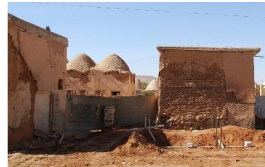
Concrete slabs over adobe load-bearing walls – © CRAterre
