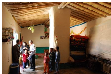
Roof with wooden structure and polypropylene screen course – © CRAterre
