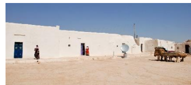
Whitewashed façades – © CRAterre
