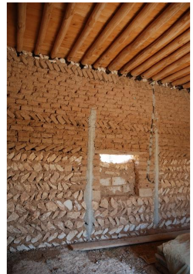
Electricity network embedded in adobe wall with cement mortar – © CRAterre
