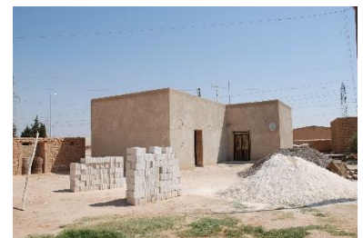
Cement-based constructions taking the place of local traditional materials and typologies – © CRAterre
