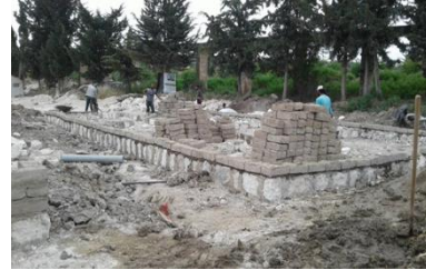
Al-Faroukia - construction site, base of the adobe walls – © QRC/BINAA
