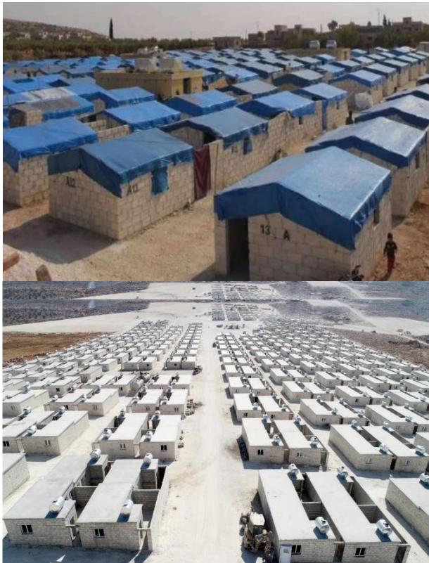
Transitional shelter: concrete block shelter – © NWS-XB-Hub Shelter Cluster
