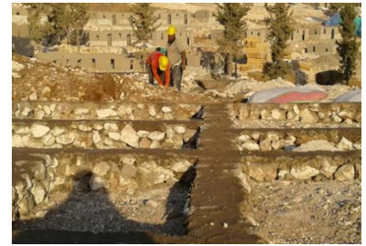
A decent life - construction site, foundations and basement – © QRC/BINAA
