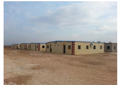
Afes – project houses in construction (top) and finished (bottom) – © QRC/BINAA
