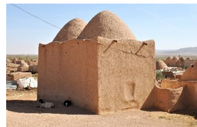
High dome with mud plaster – © CRAterre
