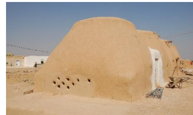
Holes left for ventilation – © CRAterre
