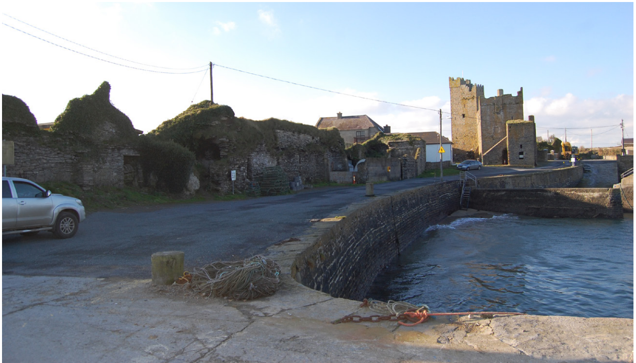
Figure 1. The 17th century salt works site at Slade, County Wexford.
