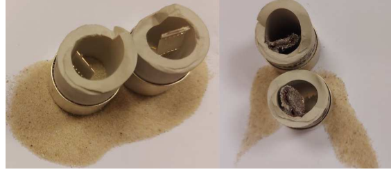
Figure 2 : Cutting of a new (left) and a blown (right) gG fuse.
