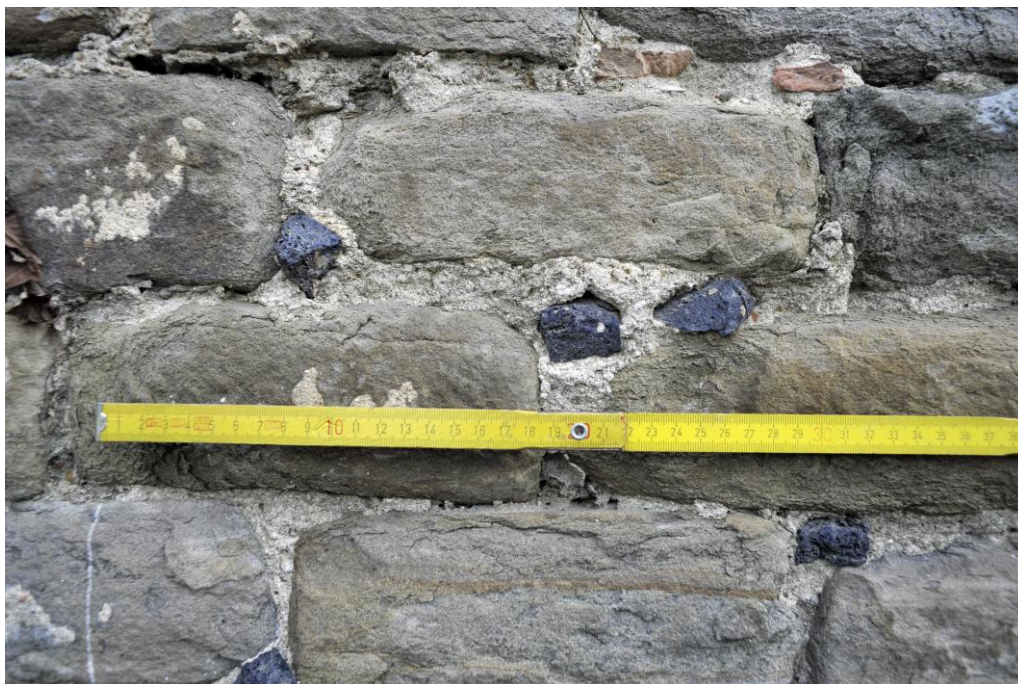
Figure 5 - Vitrified bricks present as a decorative element in the joints of the bell tower of the Pieve di San Giovanni Maggiore.
