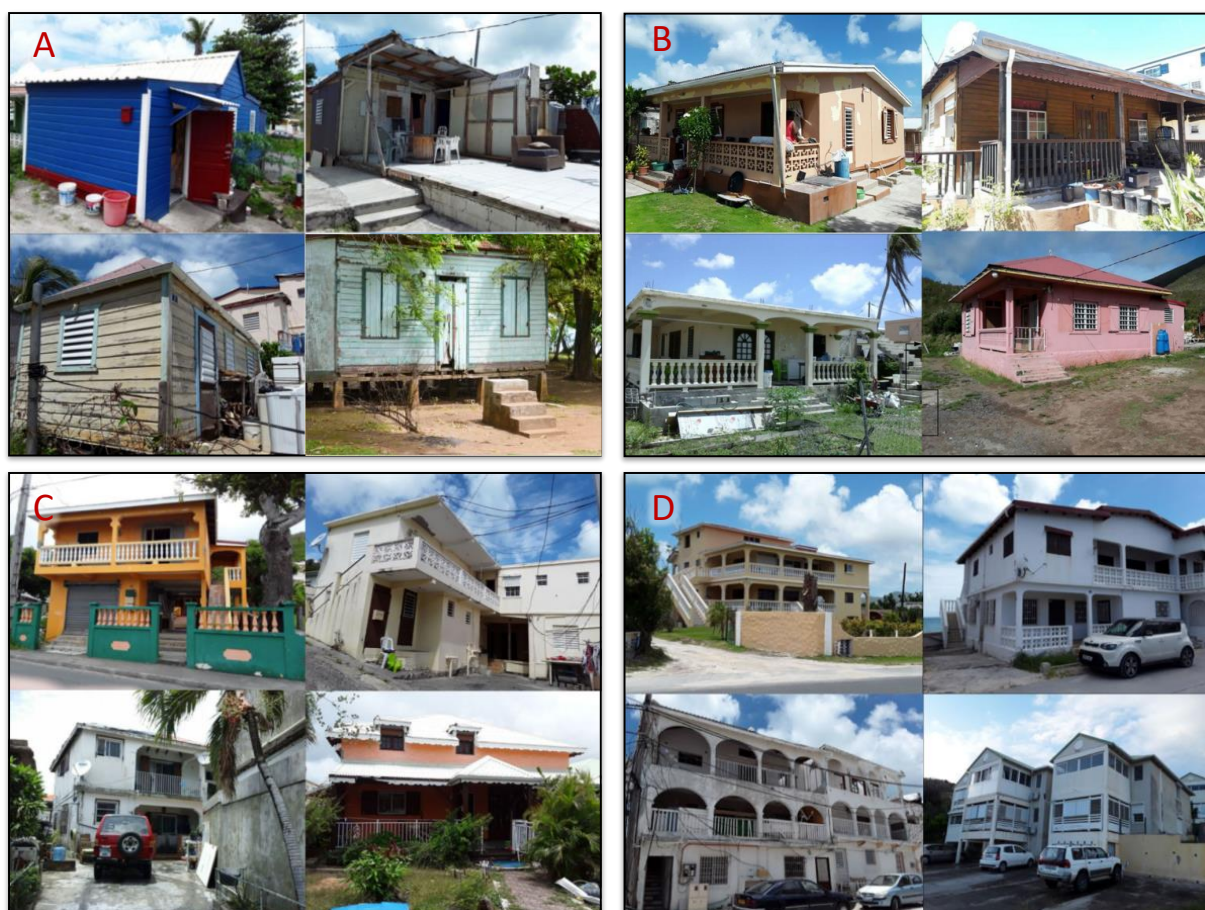
Figure 3. Different building types in St-Martin. (A): Individual dwelling without story, without masonry, in wood or sheet metal. (B): Detached single-story dwelling in masonry, stone, or reinforced concrete. (C): Individual dwelling with story(s) in masonry, stone, or reinforced concrete. (D): Collective housing in masonry, stone, or reinforced concrete.
