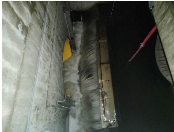
Figure 3: Photo of the outlet part of the facility during a rain event with water flowing over the filter cassette
