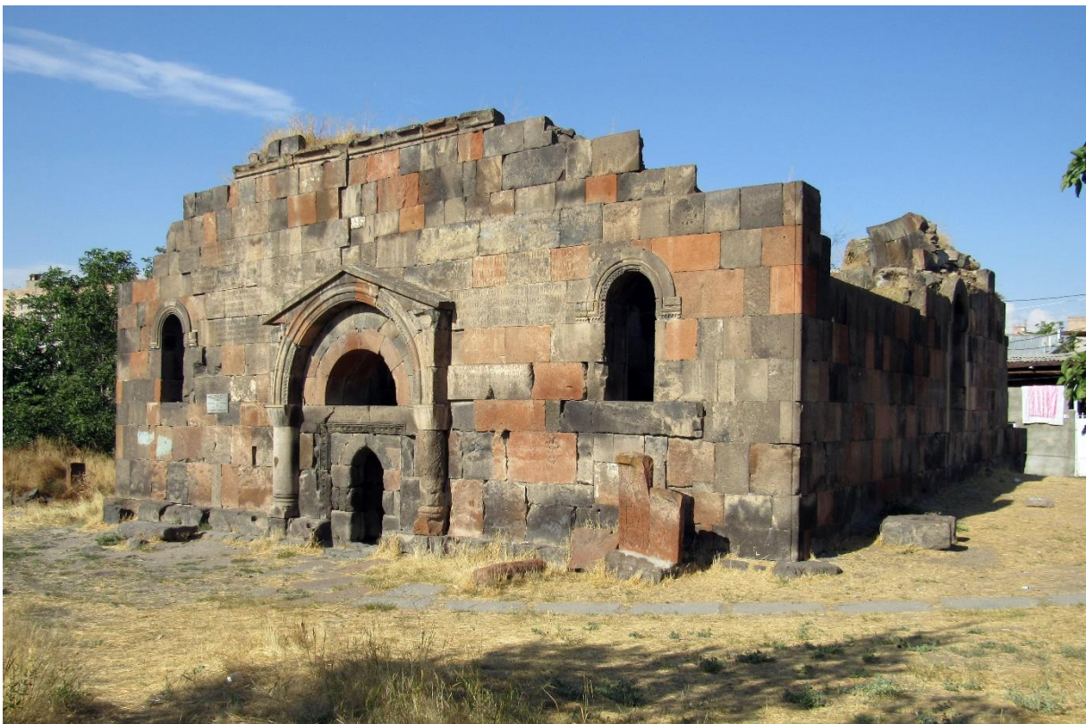
Fig. 10b. Awan Cathedral, 590s, general view from southwest © Author
