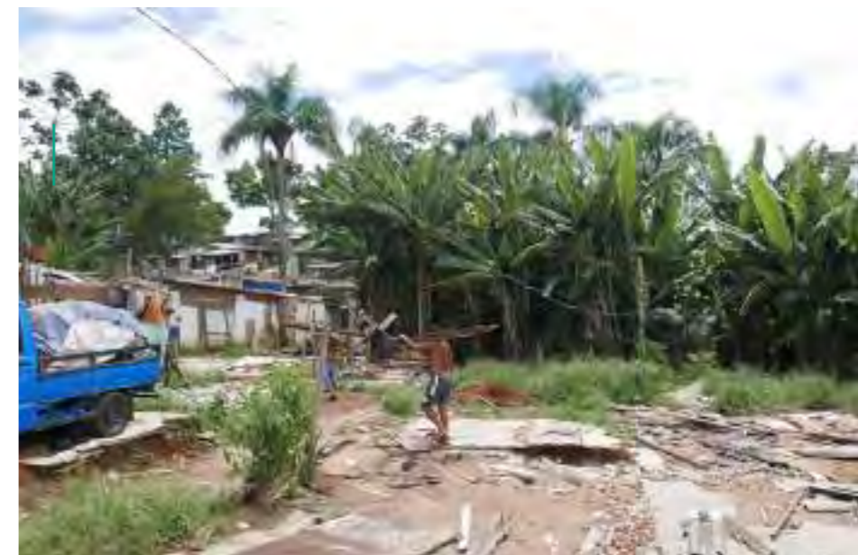
Fig.6. Process of deconstruction in protected area, Anchieta, 2020.
