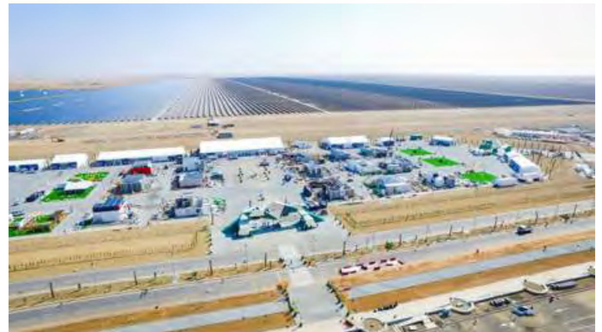
Image 1 Aerial photo of the Solar Hai, during the assembly of the teams' prototypes on site. © www.solardecathlonme.com
