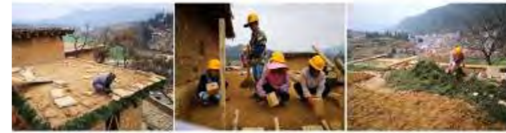
(b) Construction of Tuku house
