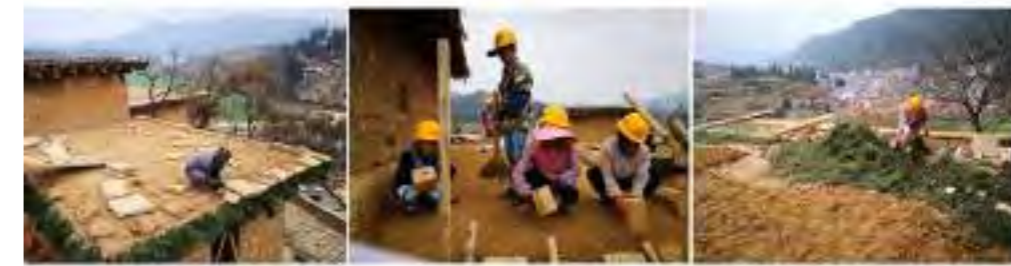
(b) Construction of Tuku house
