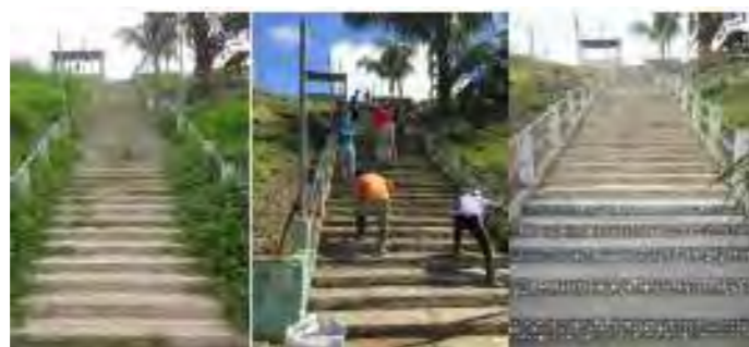
Fig. 3 Proposal for the staircases as open spaces. Betterment of the staircases. Chamanga, Ecuador. Construction: C. Mendoza, A., Koornneef, Students MICSEA 2016-17 and community of Chamanga.
