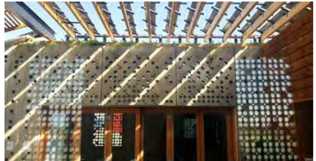
Image 6 The solar canopy with integrated photovoltaic panels, providing shade to the courtyard and preserving the evapotranspiration of the plants to achieve a local microclimate. Baitykool
