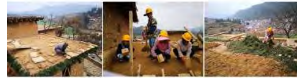
(b) Construction of Tuku house
