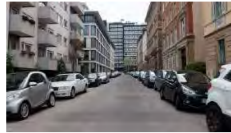
Fig. 2: Augustenstrasse in Stuttgart West, Source: Puspahati, 2021
