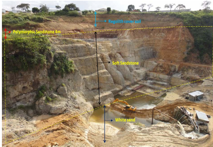
Figure 4. Macroscopic view of the lithostratigraphy section at the projected location of the Kakobola hydroelectric power plant.
