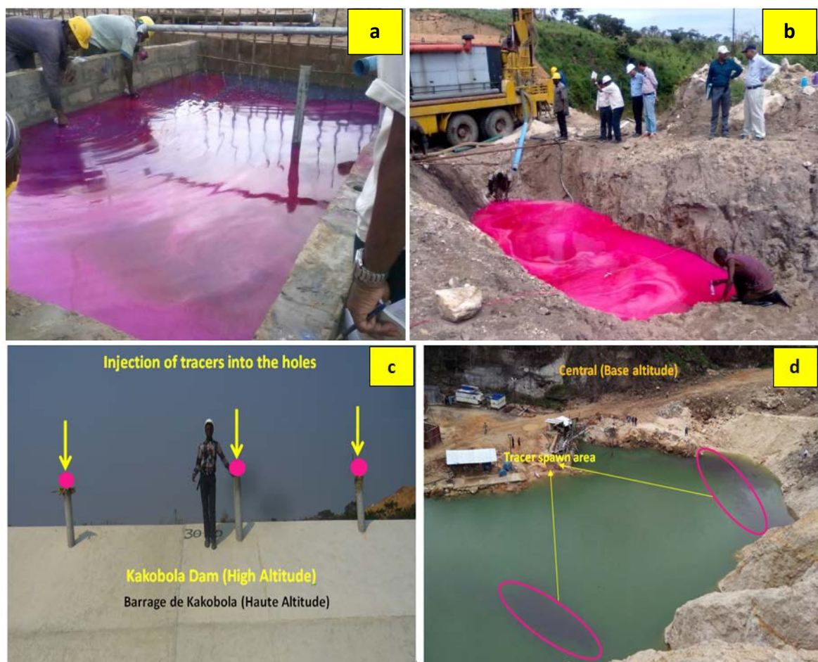
Figure 2. (a, b) Preparation of stained tracers in the Lab in blue-violet and pink in the field; (c, d) Injection of tracers into boreholes at the dam, Impact of injected tracers and appearances of tracers at the plant site through two points.
