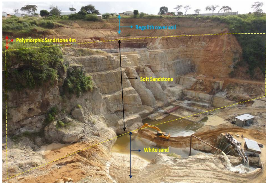
Figure 4. Macroscopic view of the lithostratigraphy section at the projected location of the Kakobola hydroelectric power plant.
