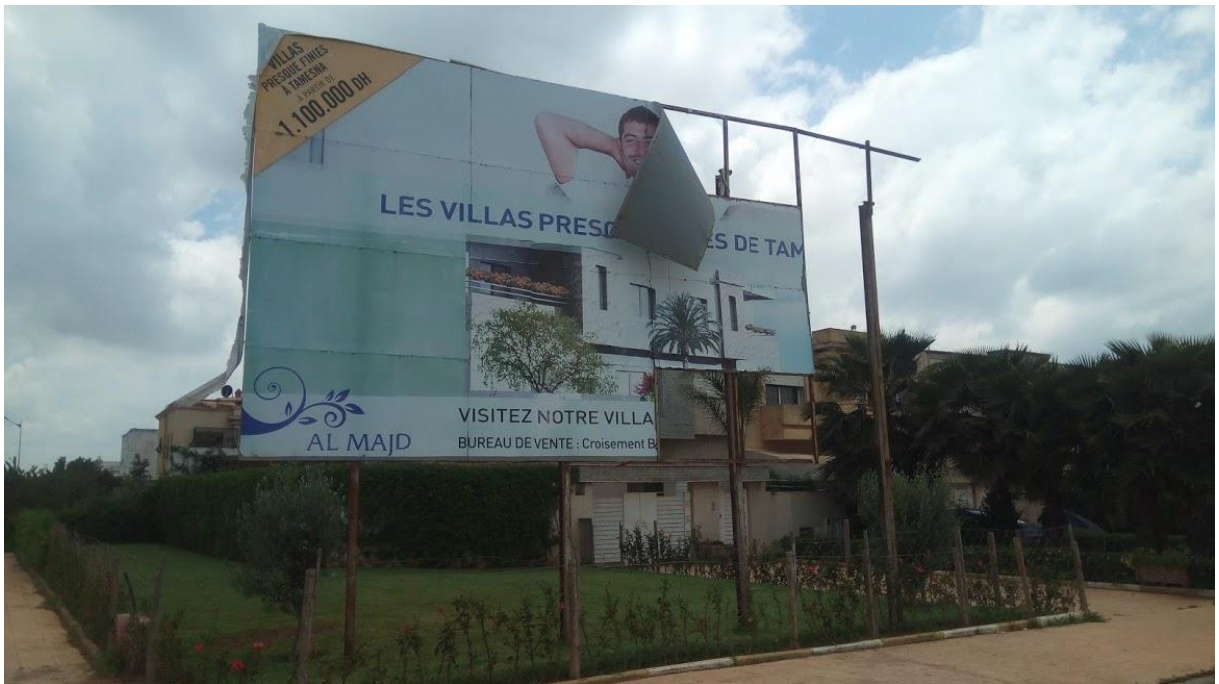
Dilapidated billboard for a villa development, Tamesna new town, Morocco (credit: Max Rousseau)
