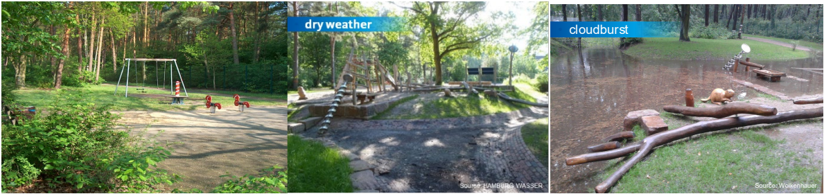
Figure 3 : pictures of the playground, left : before transformation into a stormwater playground ; middle : playground after transformation ; right : during rain event
