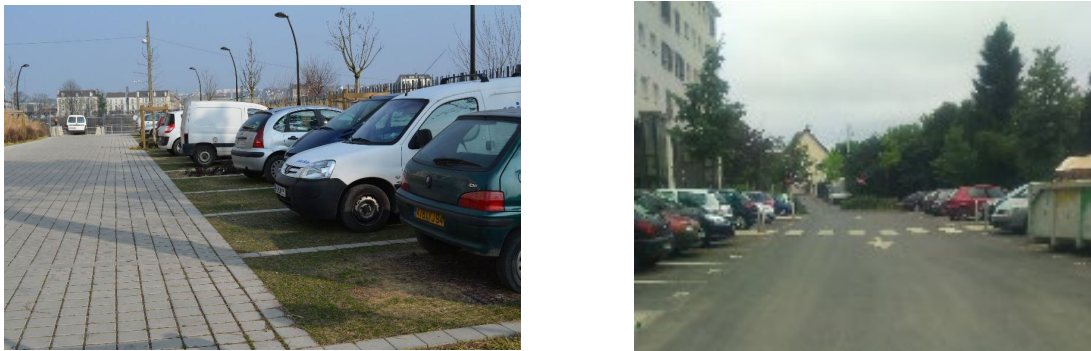
Figure 1: Photography of the studied parking lots. Left: green permeable parking lot (PP). Right: reference parking lot (PRef)
