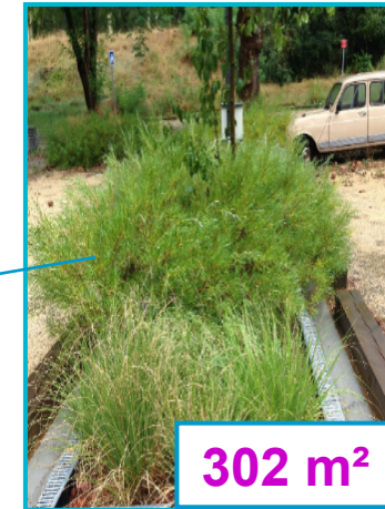
Vegetated Infiltration Swale
