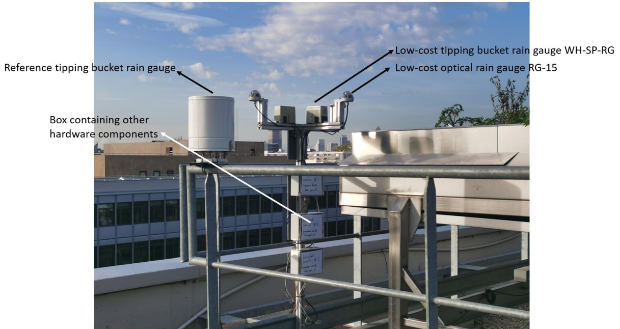
Figure 2. Low-cost rainfall monitoring stations installed on the GROOF platform.
