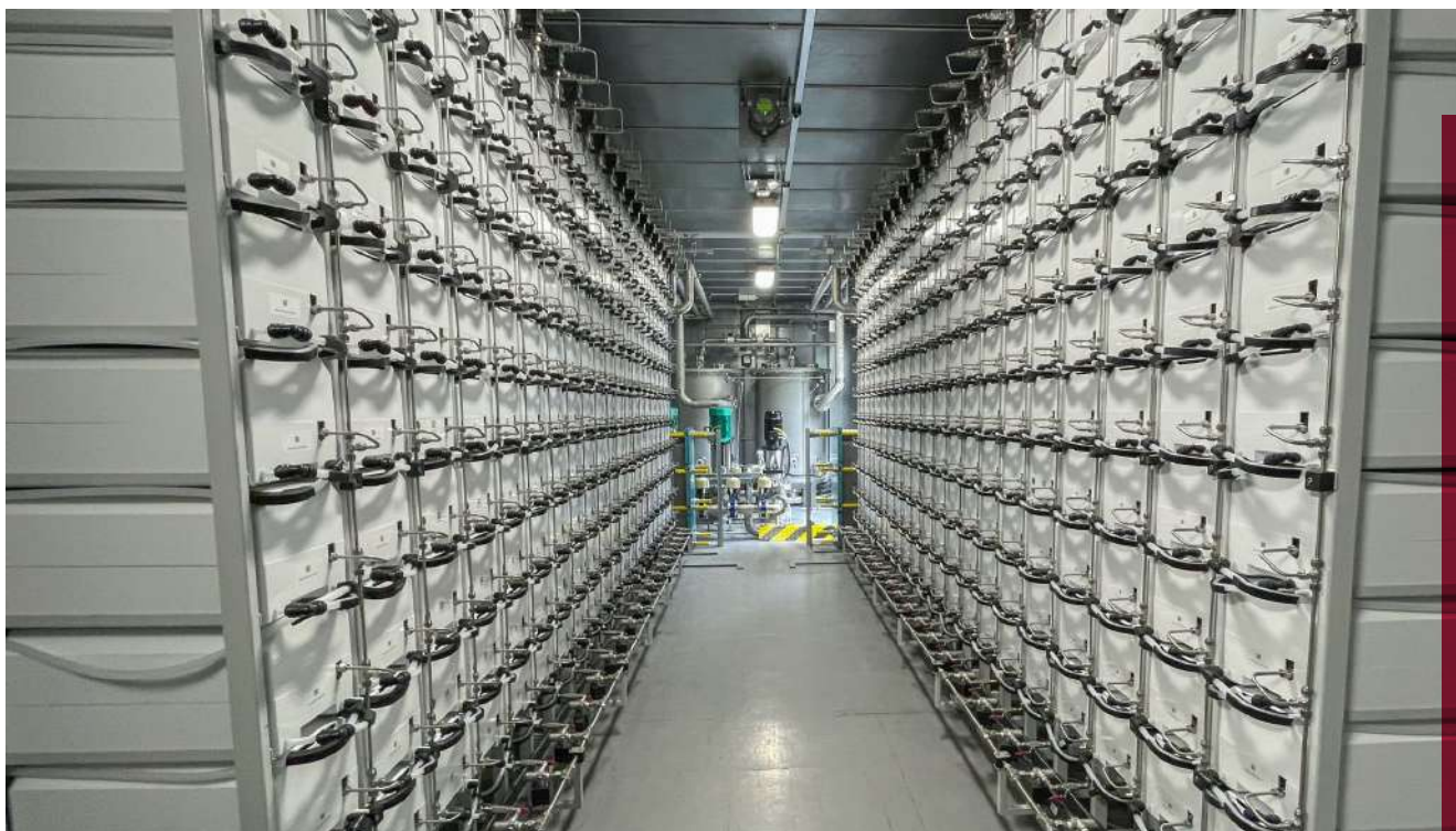
Enapter world's first megawatt-class AEM electrolyser composed of 420 modules (450 kg H 2 /day), North Rhine-Westphalia, Germany, May 2023 (Courtesy of Enapter)
