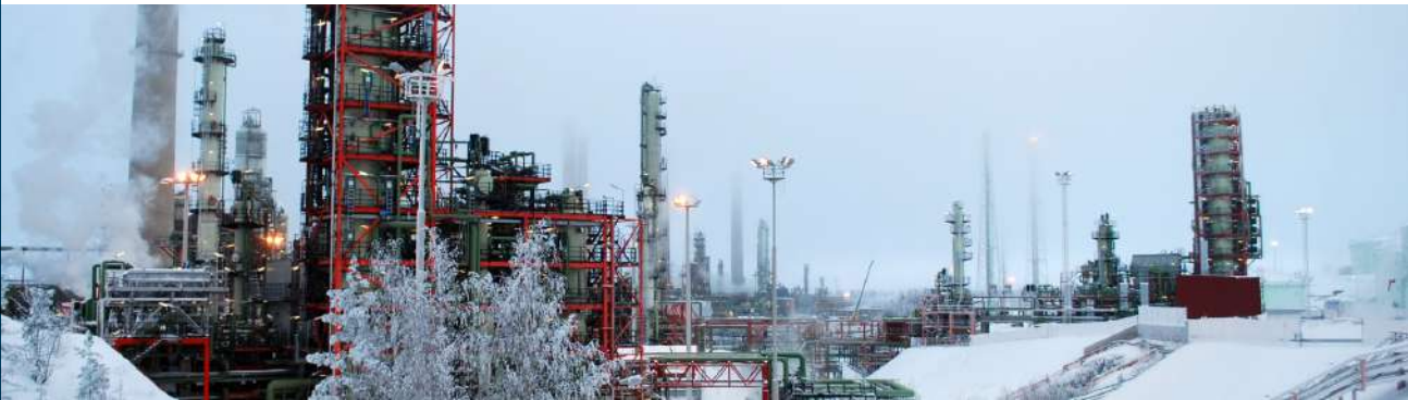
Neste's Porvoo refinery in Finland, where the SHARC project funded by the EU Innovation fund and aiming to produce hydrogen from natural gas with CCUS (along renewable hydrogen from water electrolysis) will be built (courtesy of Jobsite)
