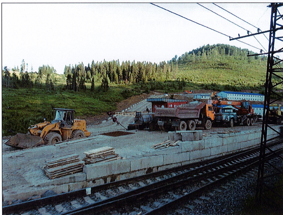
Photo 3. Construction of the new Beskydskyi tunnel
