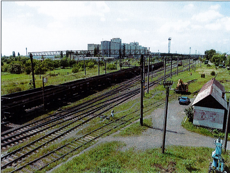
Photo 2. The modernised freight station of Uzhgorod II
