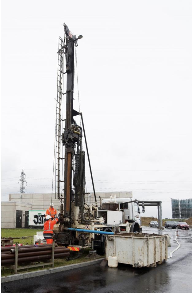
Figure 2: Core drilling. Photo: Per Lindh.
