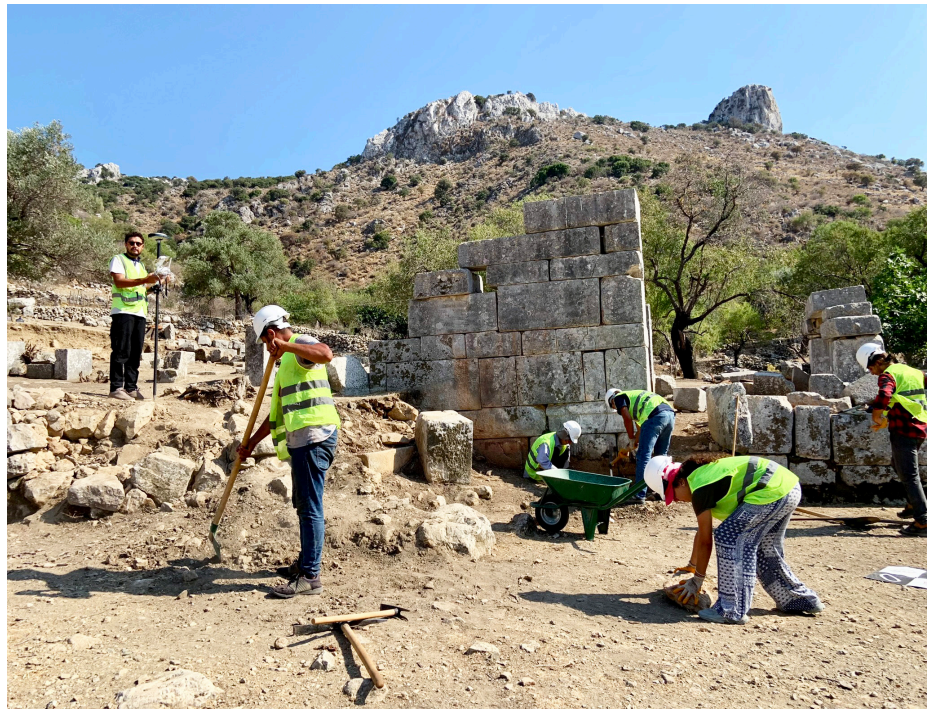
Excavation and landscaping. Photo: İlayda Alikaya
