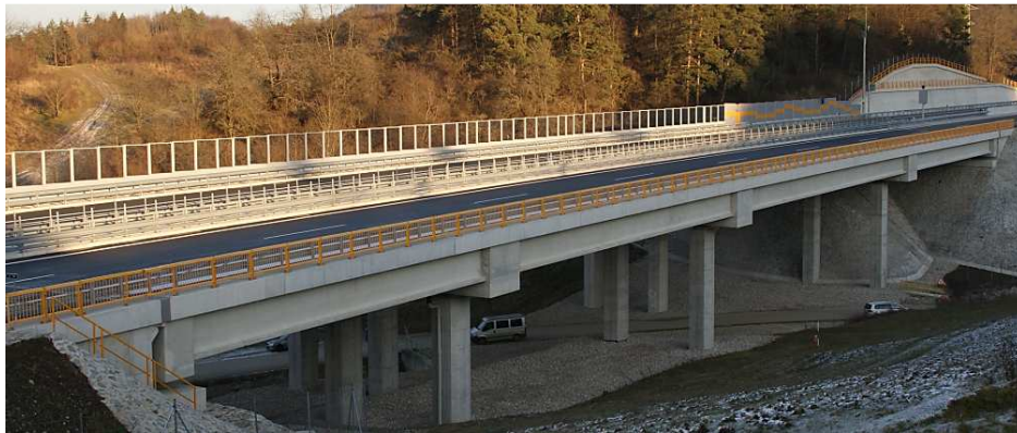
Fig. 3: View on analysed precast girder bridge.
