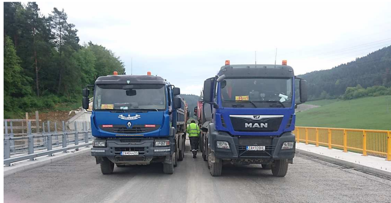
Fig. 10: Proof-load test in Span No. 4.
