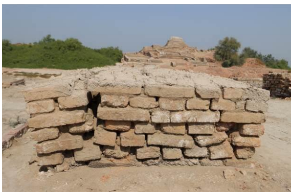
Two column types of wall (L and DKG areas) illustrating well the typical collapse process starting from the base
