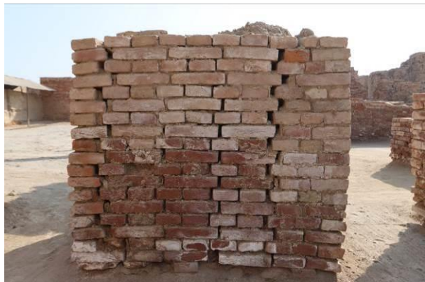
Structural cracks allowing infiltration and salt dissolution
