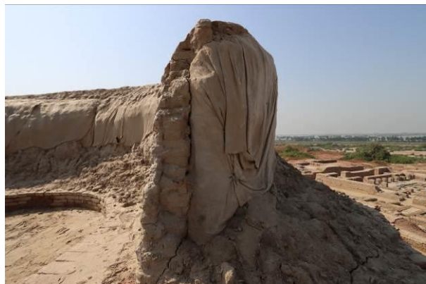
Picture showing fallen part and protective geotextile
