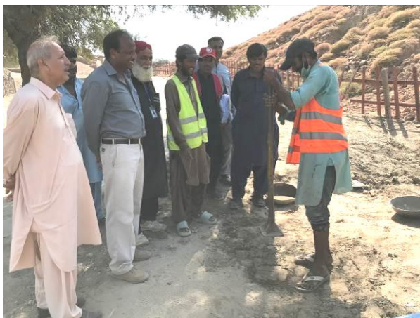
Successful repair of a gully at the entry of SD area
