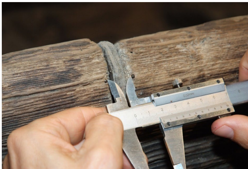
Manual measurements between sections
