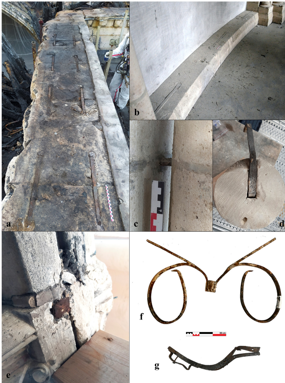
Fig. 2. Iron armatures in Notre-Dame de Paris. (a) Cramps discovered on the top of the upper walls (b) cramps in the tribunes (c) & (d) cramps attaching monolithic columns blocs to the piers in the nave (e) ancient iron bars remains in the upper bays (f) iron armature of lead cresting (g) iron armature of spire lead decoration.
