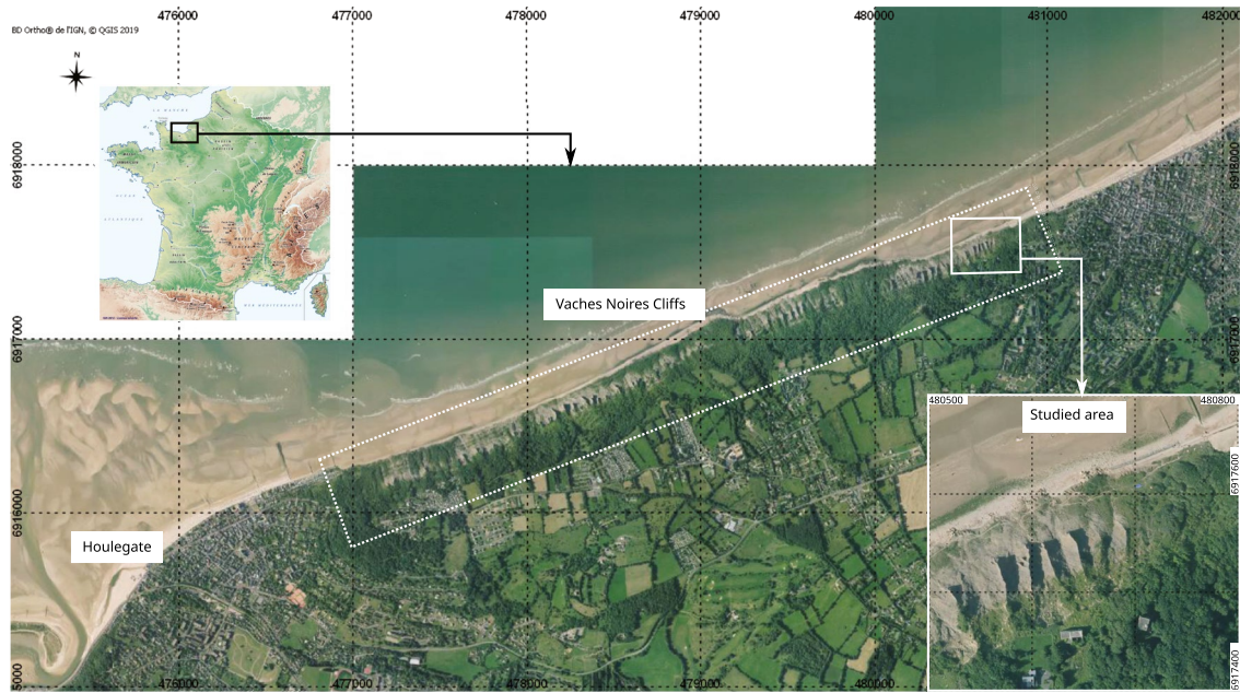
Fig. 1 Aerial view of the whole 4-km-long VNCs between Houlegate and Villers-sur-Mer (Normandy, France, white-dotted rectangle). VNC case study is encircled in white rectangle (Image from ©IGN inside ©QGIS)
