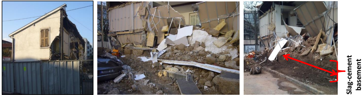
Figure 1 : Collapse of a rammed earth structure with 11%-13% water content in the walls
