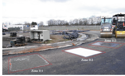
(a) 25 m track with artificial defects before laying the wearing course layer. 'Zone 113' indicates Tack-free based defects (Zones 111 and 112 are respectively Geotextile and Sand-based defects)
