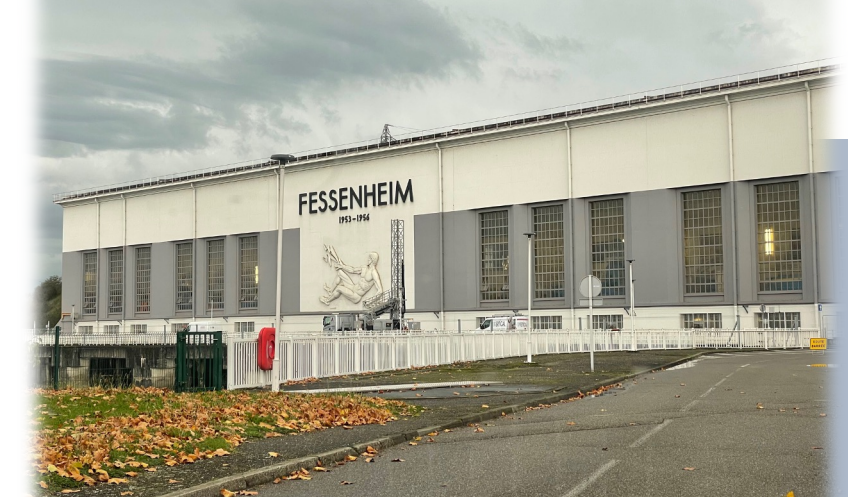
Hydroelectric dam on the Rhine River
