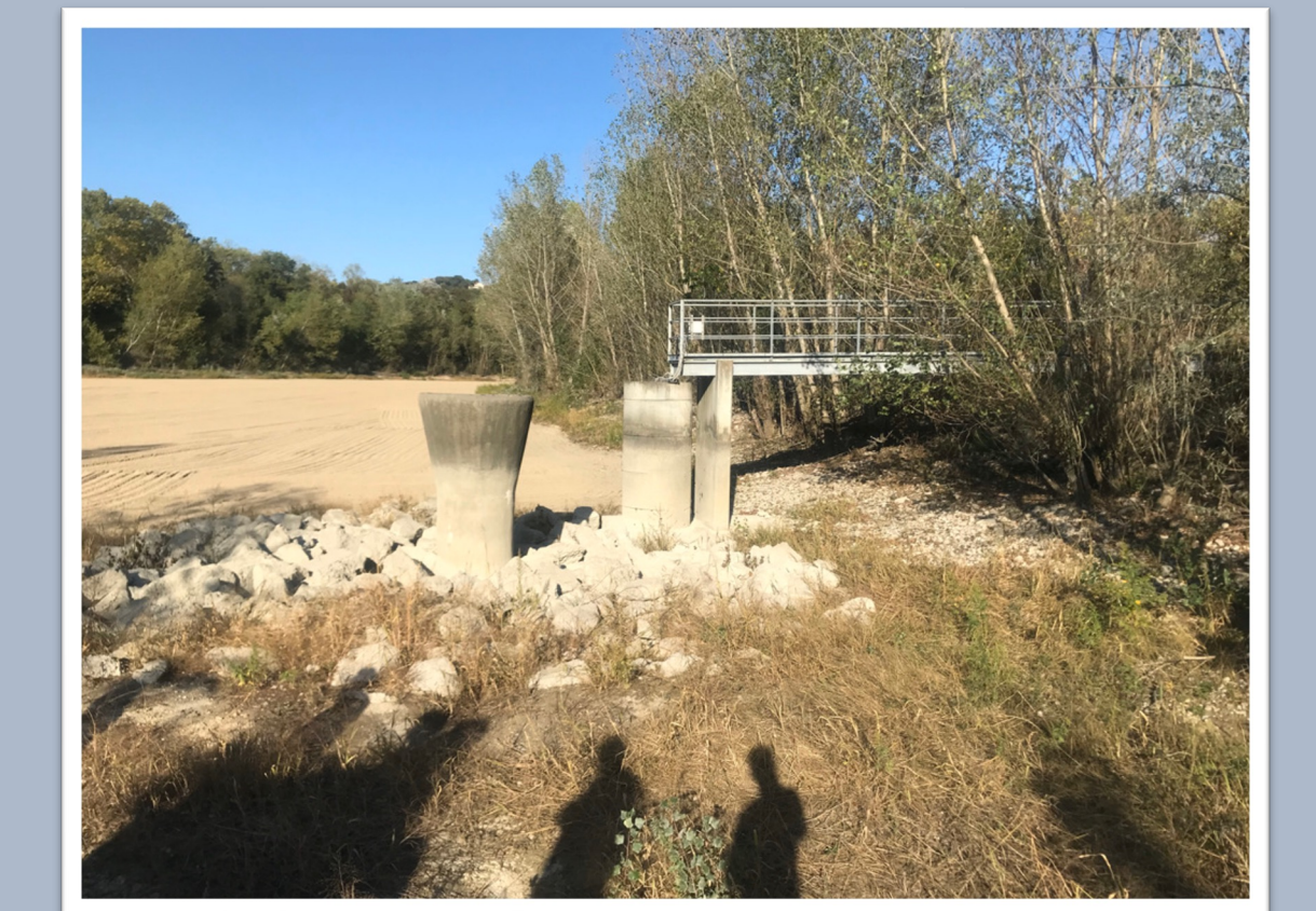
Wellfield of the Crépieux Charny water production facility (Lyon, FR, September 2019)
