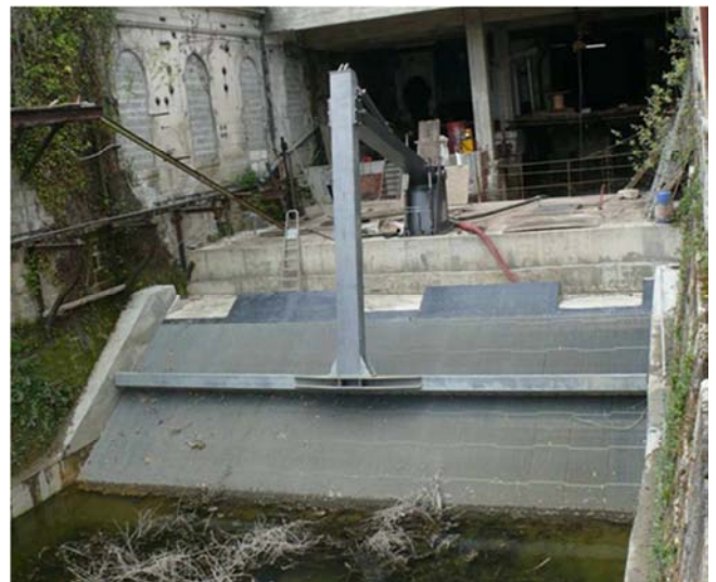
Figure 1 : Existing inclined trashrack with three bypass entrances and with cleaning equipment (Monfourat, Dronne). Photo by O. Guerri.
