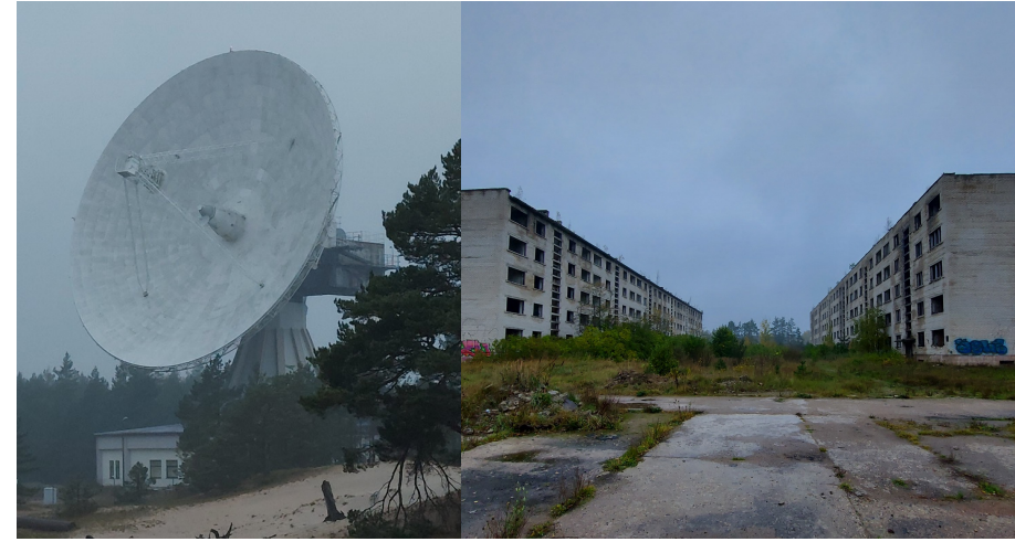
Example of former military infrastructure on the Latvian coast
