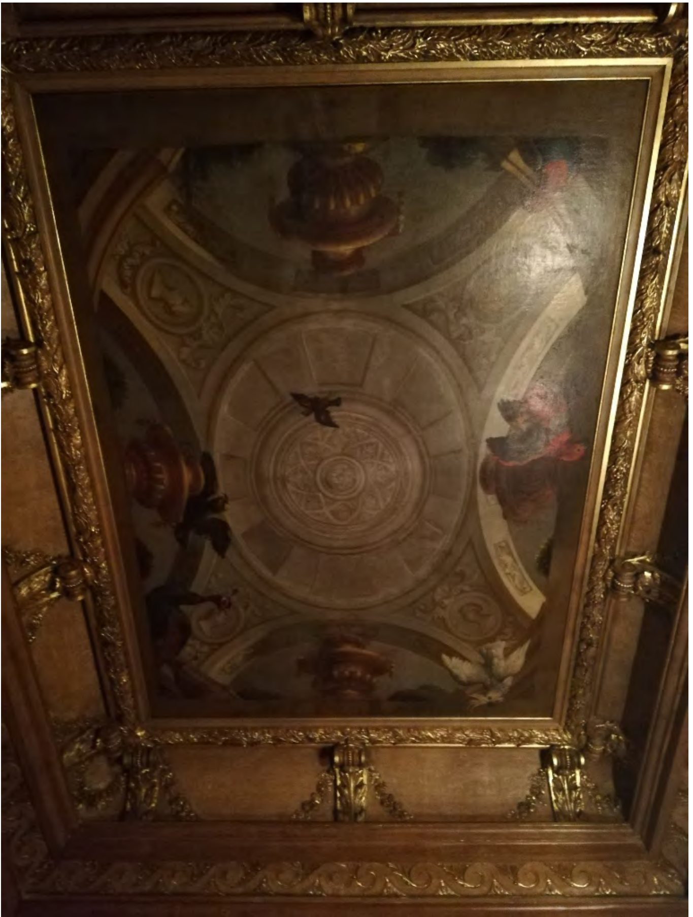
Figure 18 Photography of the plafond à curiosités on the second floor's rear building of the Hôtel de Lauzun, Paris, 2019 (author's photo).
