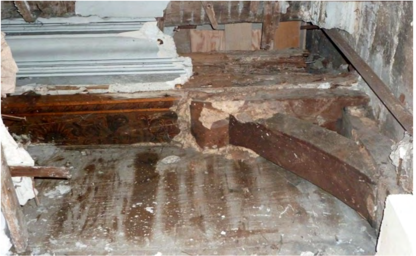
Figure 17 Jean-François Lagneau, photography of the sondage of a plaster ceiling in the rear building of the Hôtel de Lauzun, Paris, 2012 (Institut d'Études Avancées de Paris, DDOE).
