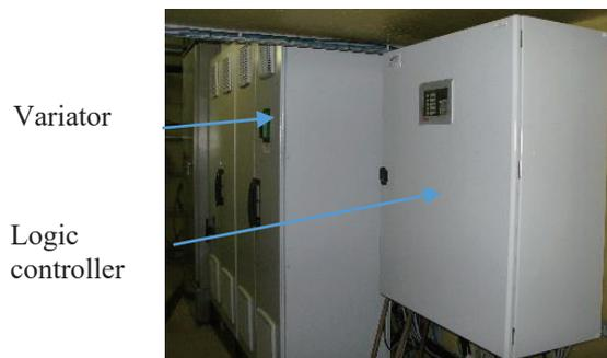
Fig.5. Frequency variator and automate installed in the pit.
