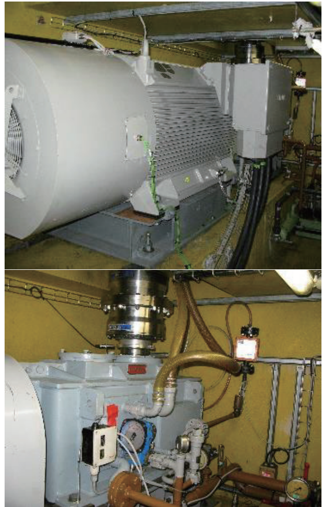
Fig.4. New engine (top) and remaining gear box (bottom) in the pit.
