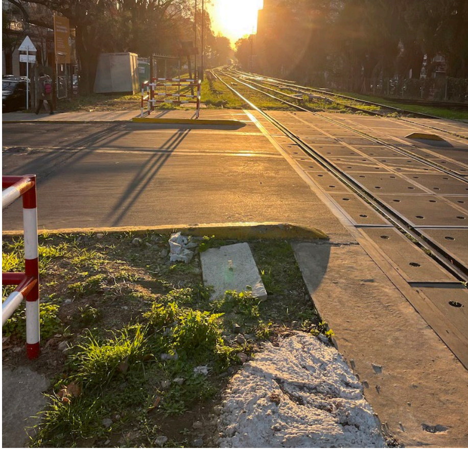
Image 17: a railway crossing in Buenos Aires. A critical infrastructure to rediscover.
