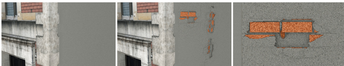
Fig. 1. A building with deep weathering effects. Left: the original building. Middle: the same building after the simulation of water particles penetrating the gray area. Right, a closeup view of the resulting degradation is due to weathering effects. Surface noise is part of the wall texture itself.
