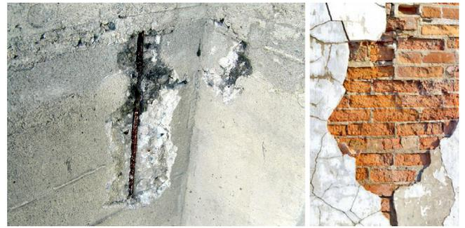
Fig. 4. Two real examples of weathering effects of water and rust on a building facade.
