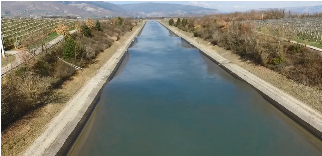
Fig. 1. View of the channel of the Sisteron dam (EDF, France). Favre waves are propagating upstream after gate closure. Photo EDF/CIH.
