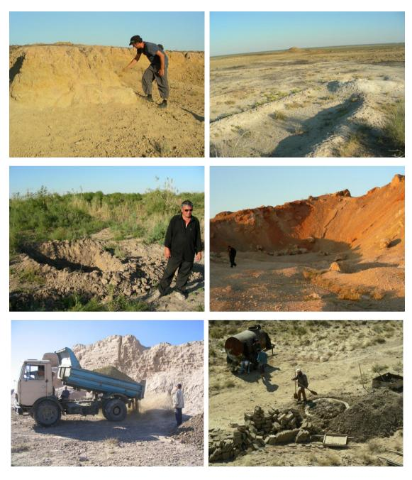
31 trucks of soil have been delivered to repair the access road and allow the circulation to the main gate of Ayaz Kala 1. 6 trucks of brown soil and 6 others of green soil, 10 water tanks, about 2000 mud-bricks of different sizes, gravel, straw and all the equipment and tools were then brought directly the conservation site.
