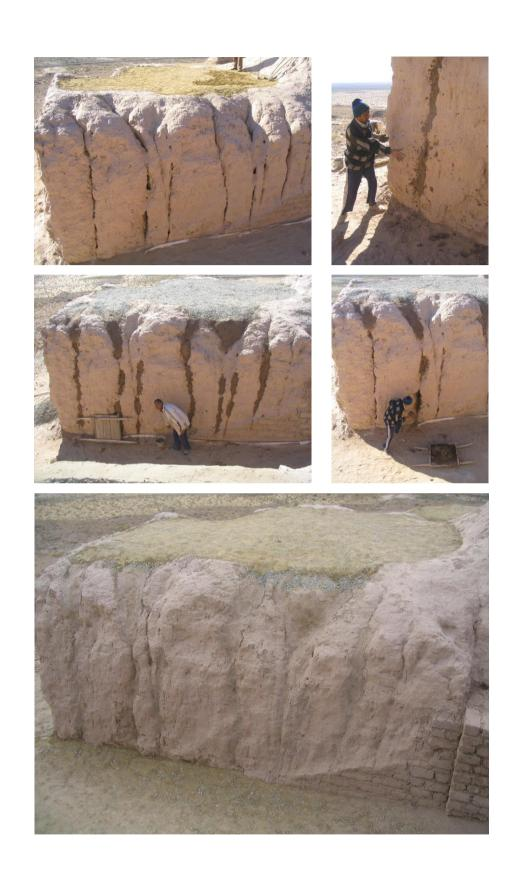
South rectangular tower Application of soil mortar as sacrificial layer on gullies dug by the rain flows
