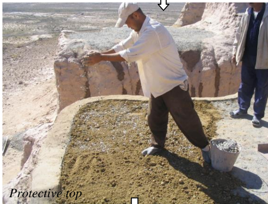
Backfilling of the tower
