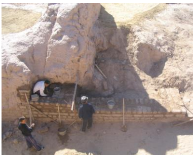
Restoration and partial restitution of the south western wall of the main gate, heavily affected by erosion. The new masonry will avoid further degradation of the original wall by channelling the water flows away from it
