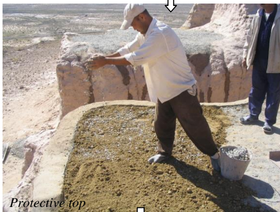
Backfilling of the tower
