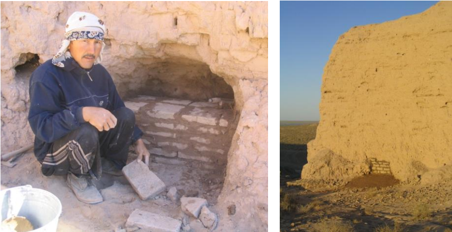
Sample reinforcement of standing walls
