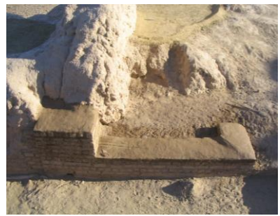
Restoration and partial restitution of the south western wall of the main gate, heavily affected by erosion. The new masonry will avoid further degradation of the original wall by channelling the water flows away from it
