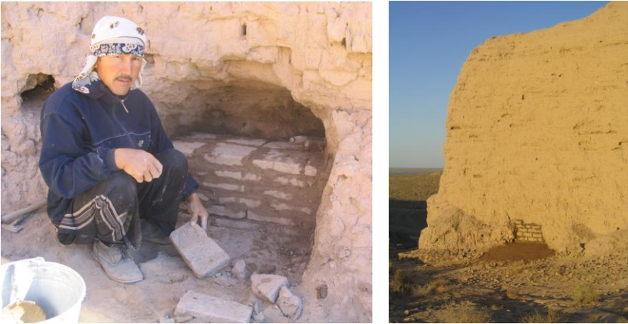
Sample reinforcement of standing walls
