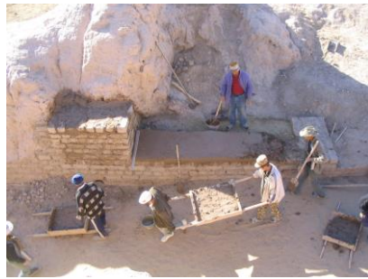
Restoration and partial restitution of the south western wall of the main gate, heavily affected by erosion. The new masonry will avoid further degradation of the original wall by channelling the water flows away from it
