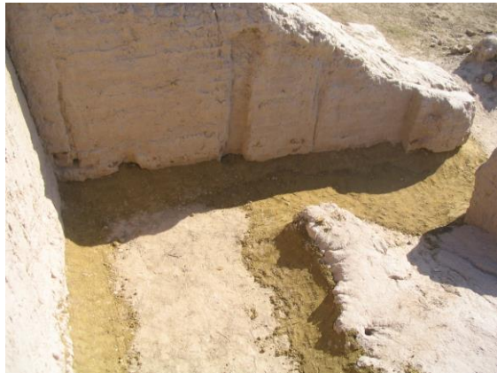
The preventive conservation techniques of superficial drainage were also employed on the remains of the temple
