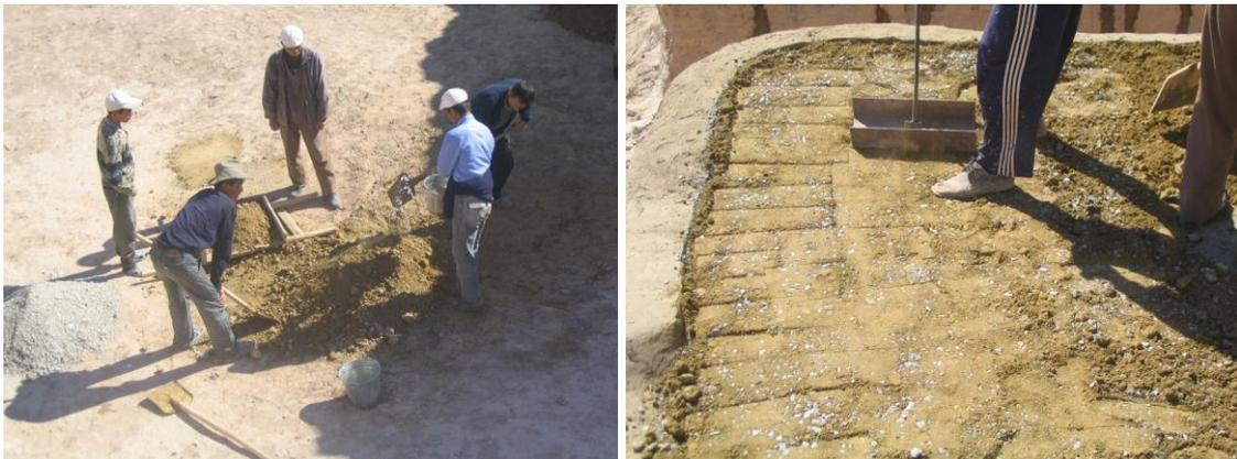
Plastering for Ayaz Kala (outside): After one week, the soil mixed with water and straw starts to smell moisture. This attention given to the soaking period has permitted to avoid the apparition of cracks which occurred with the first tests done with soil mixed with water for only one or two days.
