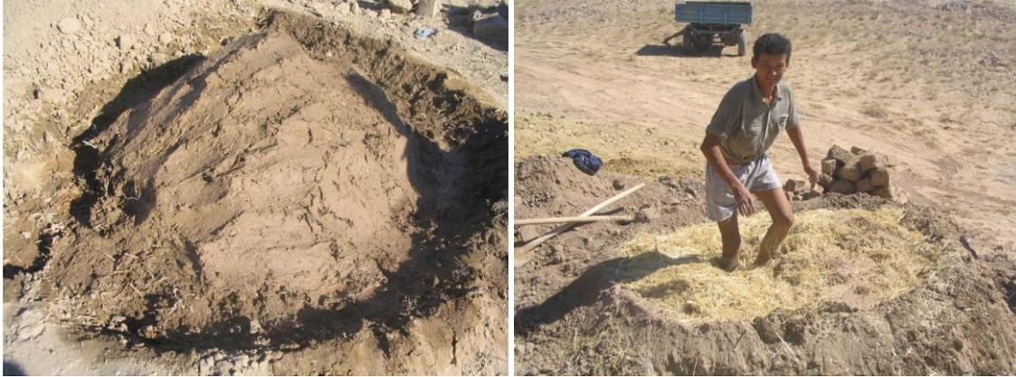
Rammed earth: Tests have been developed with a soil green in colour found 3 km at the east of Ayaz Kala which appeared to be gravelly. The results are quit efficient after ramming. Gravels have been added on the surface to reduce the speed of erosion due to rain waters.
