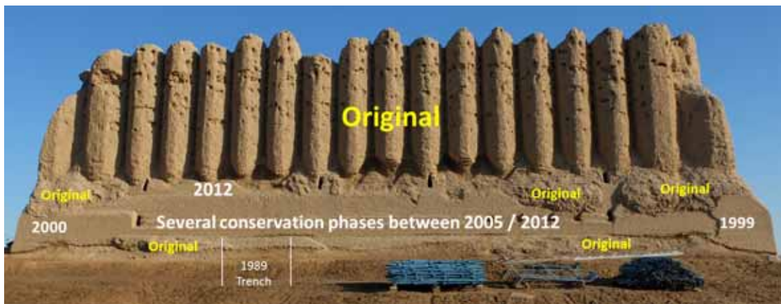
Original / Restored parts of the south facade
