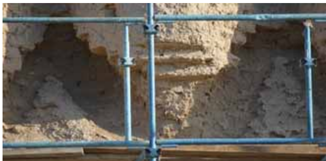
Detail of the erosion (column 10)
