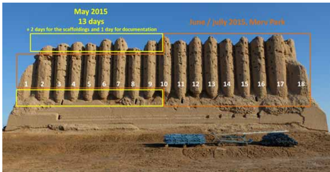
Recommended work plan for the south facade, from May to September 2015
