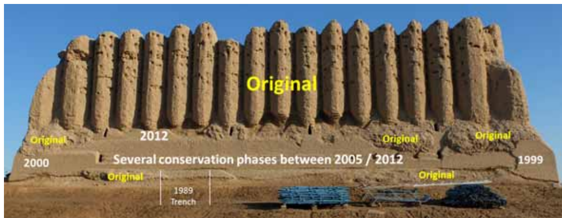
Original / Restored parts of the south facade
