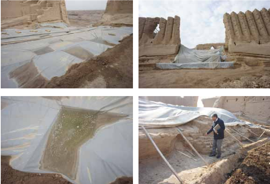
Observation of the protective textile laid on the excavated areas. January 2015
